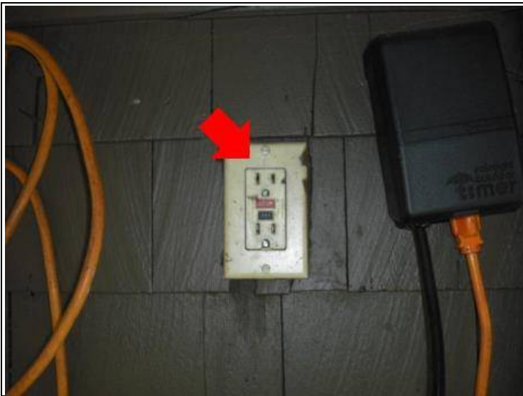
Internal GFCI's with no weather proof covers are in use externally.
