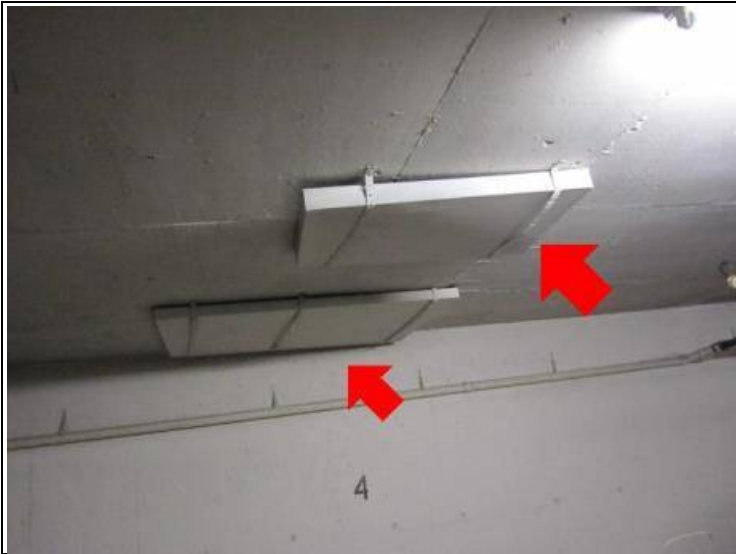
Trays have been affixed to the ceiling to collect water.
