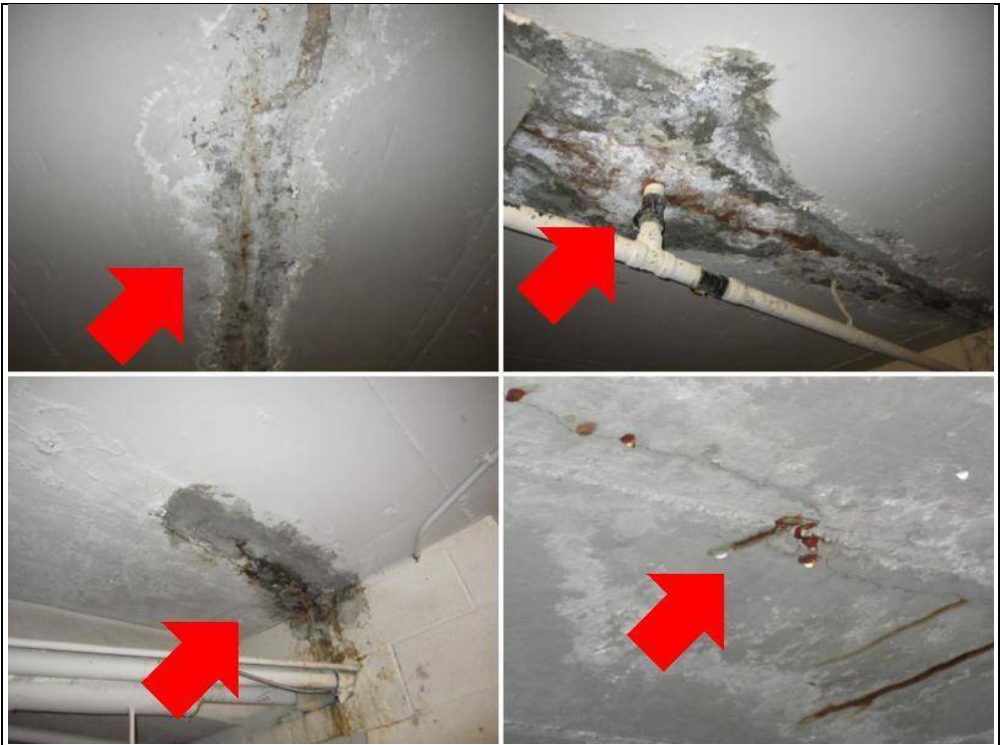
Efflorescence and water droplets were visible on the ceiling and walls of the parkade.
