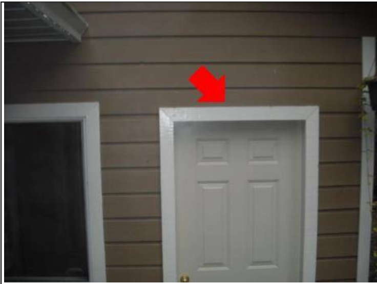
Flashings are missing on the external doors.
