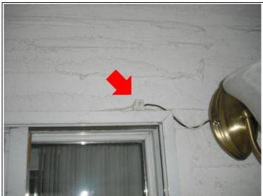
Action Necessary -An unprofessional electrical installation exists, the wrong type of wiring has been used and an inappropriate connector.
