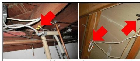
Action Necessary - I noted electrical cover plates missing, disconnected wires, untidy electrical installations etc that require the attention of a license electrician. The main areas were as follows: Basement.
