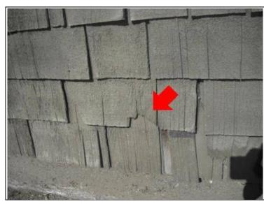
Action Necessary -The shingles are in poor condition, they are thin, split, rotting and some sections are missing. Trim:
