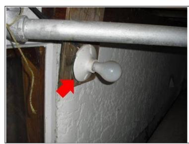
Action Necessary -At least one external light fixture is internal grade and should be changed.
