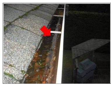
Action Necessary -The gutter system on the roof edge are inadequately sloped to carry the water to the downspouts.
