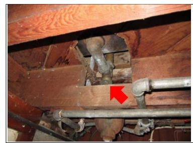
Action Necessary -At least one joist has been weakened by a large notch/hole.
