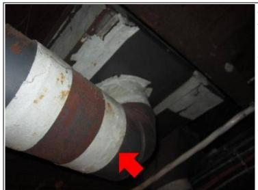
Attention Needed -Asbestos containing material was visible on the ductwork. It was commonly used on ductwork, around heat registers and as separators between ductwork and wooden framing. It is acceptable to leave asbestos in place provided it is not disturbed. However, if it
