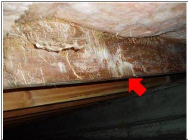
Action Necessary -Fungal growth was visible on several joists. The joists are located towards the rear portion of the basement (where the external soil level is particularly high).
