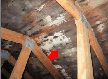
**Action Necessary -**There either is or has been a moisture problem in the attic that requires attention. This is evidenced by staining on the underside of the roof sheathing and on the trusses/rafters and rusty nails where they penetrate the sheathing. It is strongly
