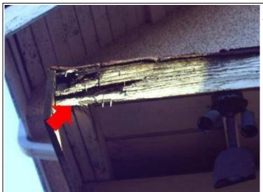
Action Necessary -The fascia & barge boards are rotting and the rot has affected the roof sheathing and the ends of the rafters. Repairs or partial replacement is needed.
