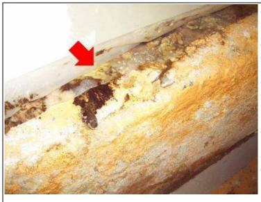
Action Necessary -Due to the high soil levels sections of the perimeter wall framing were rotting. Most of the framing was not visible due to being partly concealed by drywall. However, fungal growth could be seen growing out from the wall down the surface of the inside of the concrete foundation
