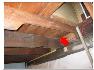
Action Necessary -Large notches/holes have been made in some of the joists which has weakened them.
