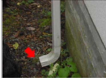
Attention Needed -Some downspouts are not discharging their run-off water correctly. Run-off water needs to flow away from the side of the building at least 6 feet. This will allow the run-off to get far enough away to not interfere with the foundation. Alternatively downspouts could
