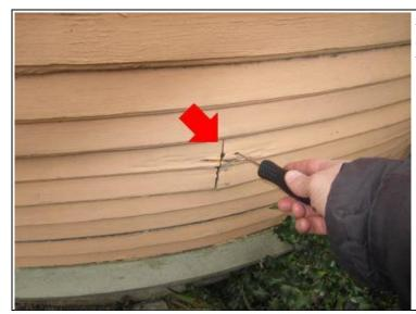
Action Necessary -Some sections of the siding are rotten.
