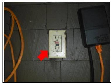
Action Necessary -An internal grade outlet has incorrectly been used outside. This requires changing as soon as possible to an external grade outlet.
