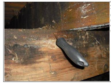
Action Necessary -The beams need repair or replacement. This is due to rotten sections.
