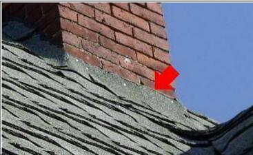
Action Necessary -The flashing installation is poor. Shingles have been merely turned up adjacent to the masonry.
