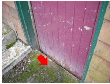
Action Necessary -There is no drain in the concrete floor of the basement walkout. This is required to eliminate or minimize the risk of water entry into the basement. Also there should be a minimum of a 4" step up into the basement from the outside (to prevent water entry).
