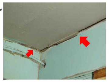
**Ceiling:** Action Necessary - there is some damage to the lath and plaster ceiling.
