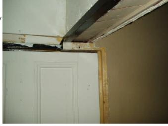
**Walls:** Attention Needed - the internal walls to this room have been poorly framed and
